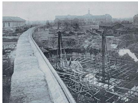
駅本屋南端(後のステーションホテル端部)の基礎工事 『東京市街高架鉄道建築概要』1914年(大正3) 用地買収も完了し高架線工事と並行して1908年(明治41)3月からは中央停車場の建設も始められた。写真中央に見える建物は明治27年に完成した東京府庁舎。 Foundation Work for Main Station Building South End (later to become part of the Station Hotel) "Summary of the Construction of the Tokyo Urban Elevated Railway," 1914 With the acquisition of land completed, construction begins in March 1908 for the Central Terminal Building, simultaneously with the construction of the elevated tracks. The building seen at the center of the photograph is the Tokyo Prefectural Office, completed in 1894.
