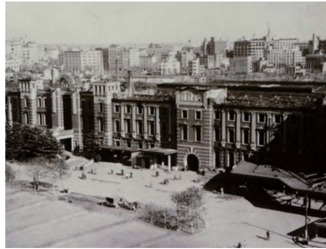
戦災直後の東京駅の被災状況 1945年(昭和20) The damage to Tokyo Station immediately after the bombing (1945)
