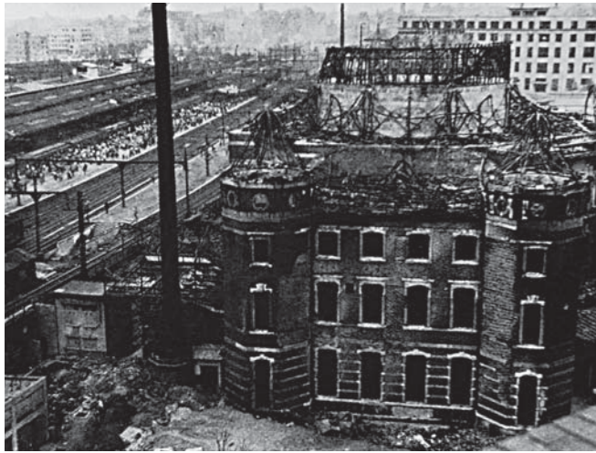
焼失した東京駅 1945年(昭和20)5月 Tokyo Station after the fire (May 1945) 昭和20年5月25日23時過ぎ、米軍B29から投下された焼夷弾により全焼、翌26日朝7時過ぎに鎮火した。象徴であった異国的な丸屋根のドームが姿を消し3階建が2階建になった。 An incendiary bomb dropped by a U.S. B29 bomber some time after 11 p.m. on May 25, 1945 started a fire that burned down the Tokyo Station Building. The fire was extinguished just after 7 the following morning. The distinctive foreign looking domes were gone, as well as the third floor, leaving just a two-story building.
