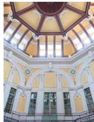
丸の内南口ドーム見上げ部分の竣工写真 Perspective view of the completed dome ceiling at the Marunouchi South Entrance
