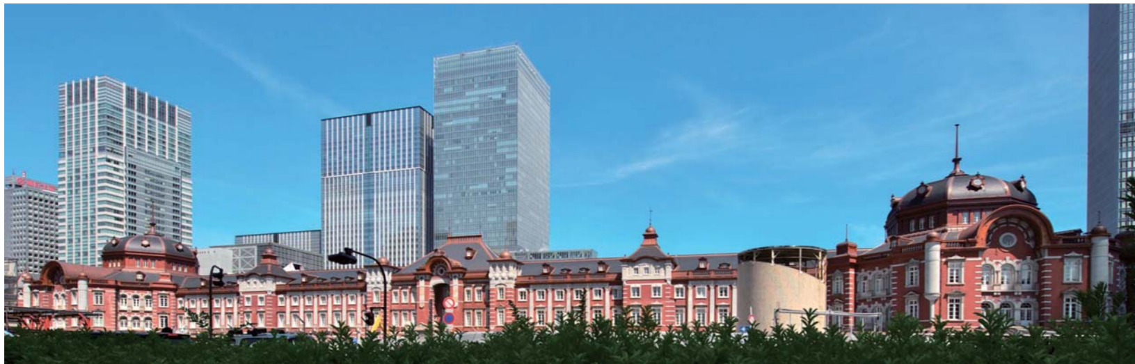
復原後の丸の内駅舎正面からの全景 Panoramic view of Tokyo Station Building front after completion of preservation and restoration work
