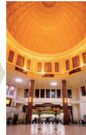
Perspective view of the dome ceiling after post-war restoration
